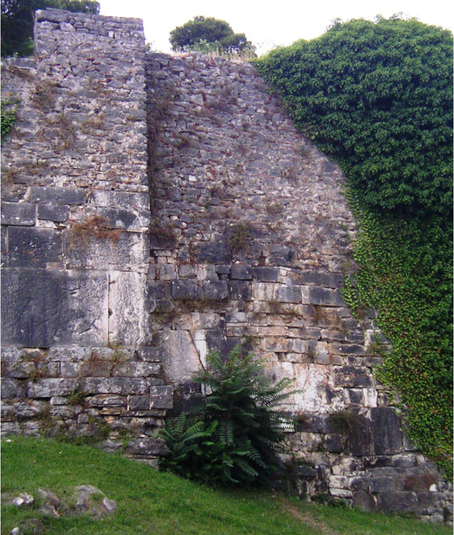
Fig. 90. Castle of Arta. Section of masonry at the W part of the enceinte.
